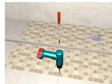
Fig. 3: Remove the channel then drill through the marked positions
