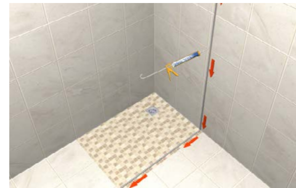
Fig. 4: Apply a bead of silicone sealant within the channels
